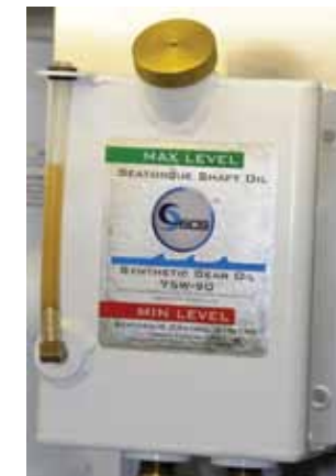
The clarity and quantity of the system's lubricating oil is easily monitored at a reservoir located above each shaft.
